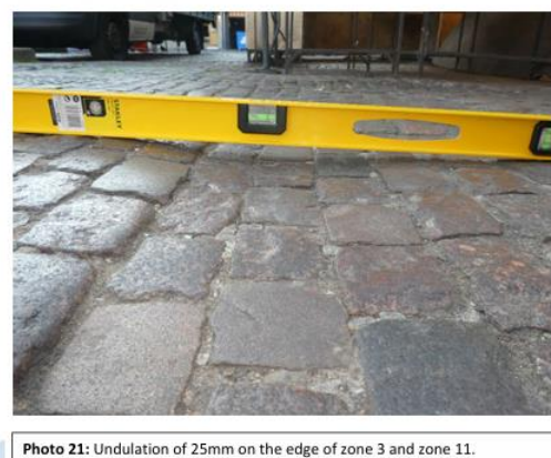
Photo 21: Undulation of 25mm on the edge of zone 3 and zone 11.
